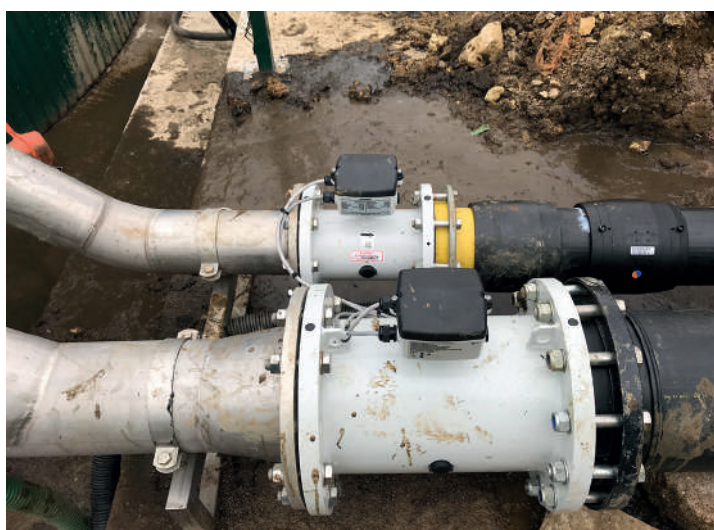
Siemens flow meters and related software and controllers have been developed by John to monitor static sites such as biogas plants. The 6- and 10-inch meters pictured on the left both patch into accurate recording software. Battery powered systems are available to service remote locations.
