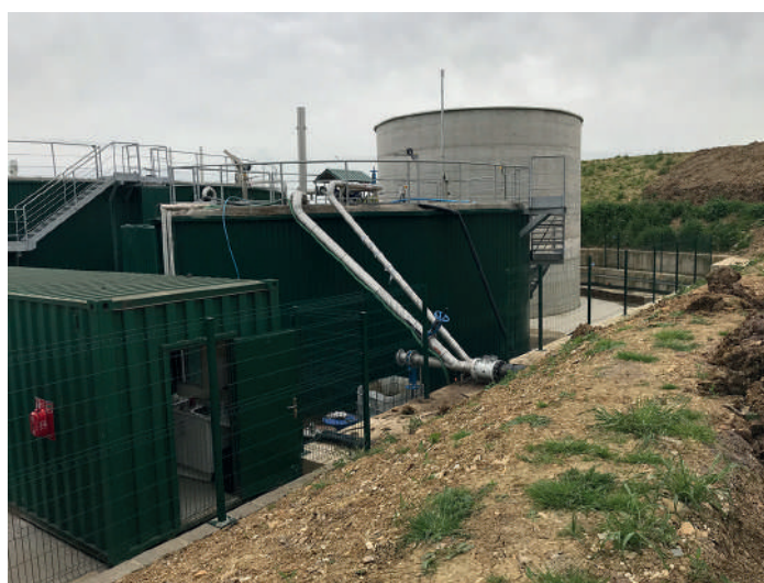
Siemens flow meters and related software and controllers have been developed by John to monitor static sites such as biogas plants. The 6- and 10-inch meters pictured on the left both patch into accurate recording software. Battery powered systems are available to service remote locations.
